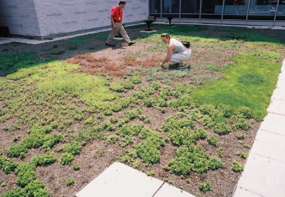
The Human Rights Campaign headquarters in the Dupont Circle area of Washington, D.C., has a 2,000-square-foot extensive green roof over the entrance gallery (above). A sign at street level (right) notifies passersby that there is a green roof located above and explains the benefits of green roofs.
