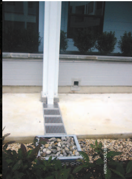
Elevation 314, a new mixed-use development in the Takoma Park area of Washington, D.C., has a 700-square-foot intensive green roof at grade over the building's parking garage, the first green roof permitted in the District of Columbia for stormwater management. Roof runoff is drained into the green roof, and excess water seeps out of weep holes into a bioretention area courtyard. A recirculating water fountain is fed by rainwater.
