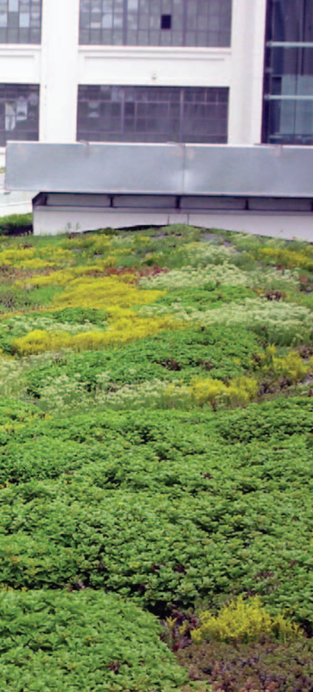
Montgomery Park Business Center in Baltimore, Maryland, has a 20,000-square-foot extensive green roof, which helped the developer to secure the lease of the Maryland Department of the Environment, the first anchor tenant, which, in turn, helped the developer's cash flow.
